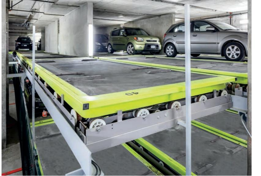
In 2015, Lödige Industries installed the first automated parking system in Ottawa. It provides parking for 47 cars in *The Eddy* building, a six-storey condo tower. The main challenge of this building was an unconventional footprint requiring a customised parking solution. The 5BY2 pallet-based technology from Lödige Industries enabled a maximum of parking slots for this unique building.
