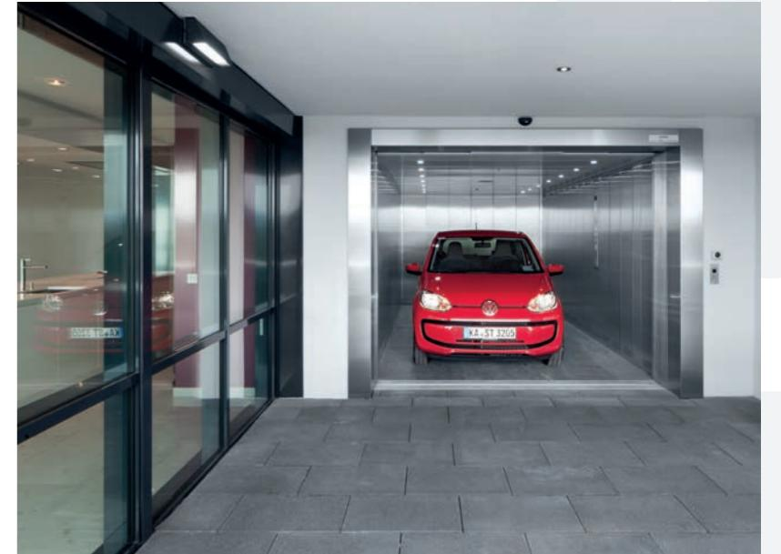
*Upper East* is a residential construction project in the high-profile Citypark development area of Karlsruhe with 145 freehold apartments, three commercial units and an underground car park. In four-story buildings, 24 of the loft apartments are equipped as so-called *CarLofts* with car lifts and loggias for parking the car on the apartment's own balcony.
